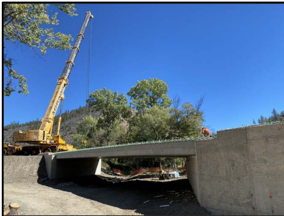
Figure 5. CNC- and Biochar-Infused Concrete Beams
