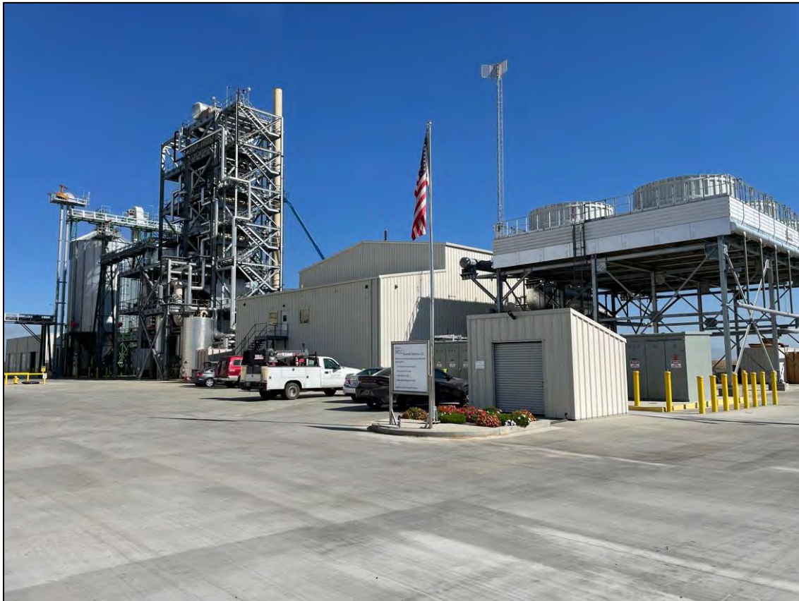
Figure 3. Biomass Direct Combustion with ORC Electricity Generation in Williams, CA
