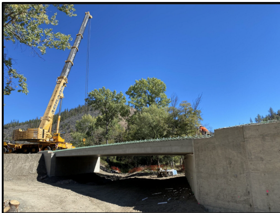
Figure 5. Nanocrystal and Biochar Infused Cement Beams
