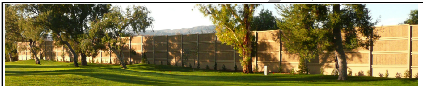
Figure 6. Wood Wool Cement Sound Wall
