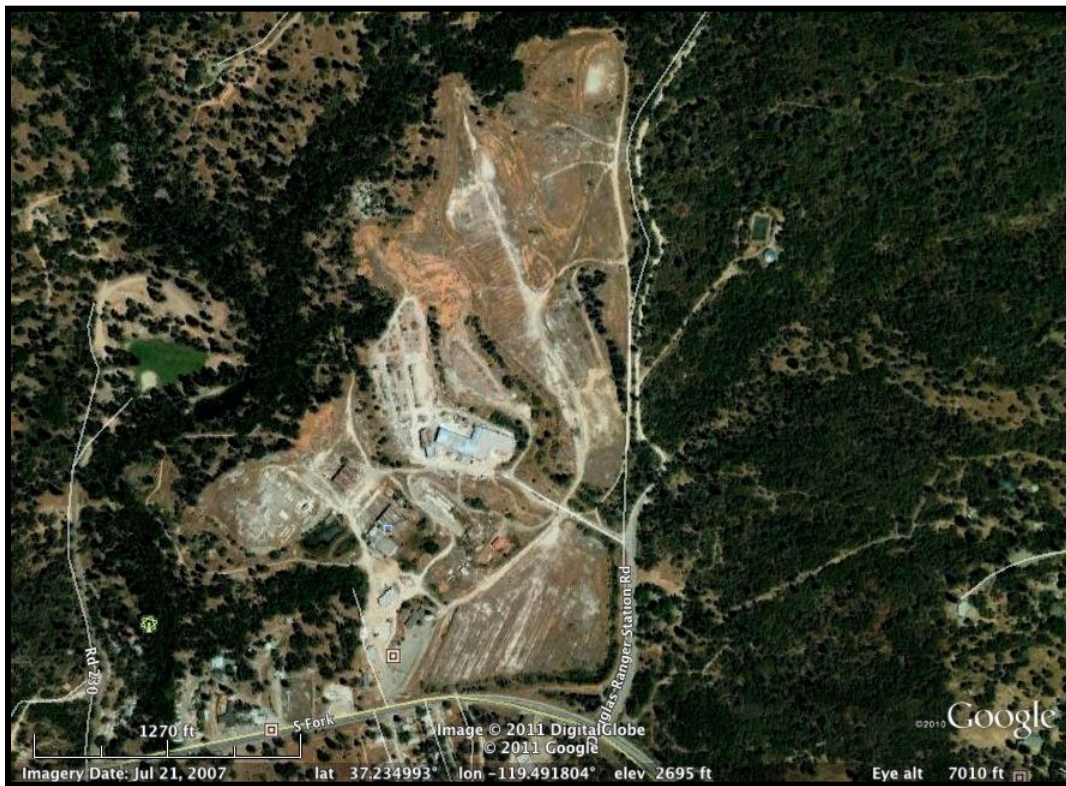
Figure 7. Aerial View of North Fork Mill Site
