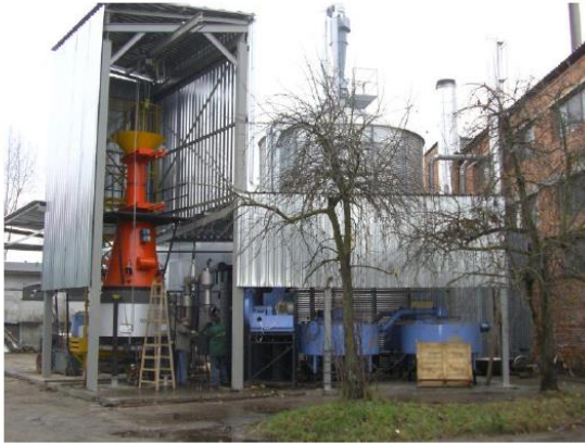
Figure 2 – The P250 biomass conversion chamber (red) and filtering system (blue)
