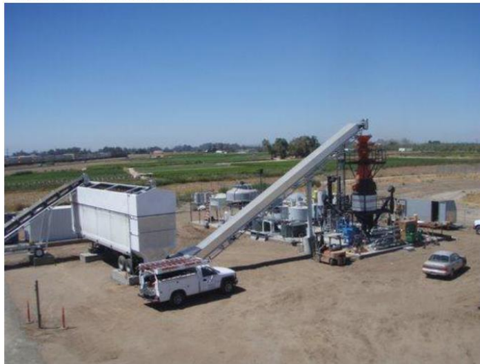
Figure 3 – A P500 installation in California
