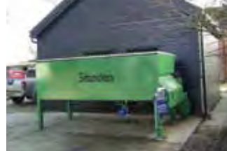
Hydraulically unloaded Storage Systems for wood chips
