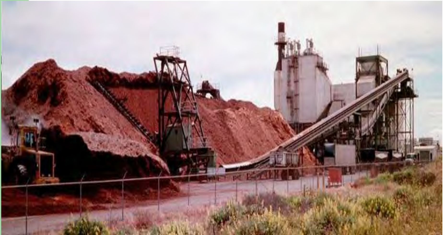
DG Fairhaven Power 18 MW CHP at Fairhaven, CA
