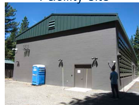
Back-up diesel generators nearby
